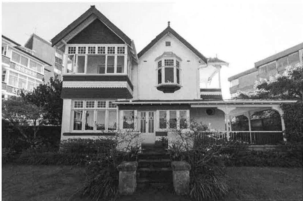
Figure 8: South elevation "Lansdowne". Note pair of gables, one roughcast with oriel window below (at right), the other timber shingled with 2-storey bay window below. Central sunroom to the ground floor is an inter-war period enclosure of part of the verandah.
