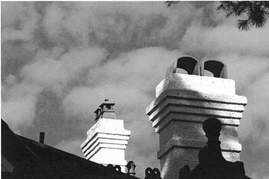
Figure 26: Chimney detail, "Lansdowne" (note two different styles of terracotta chimney pots)
