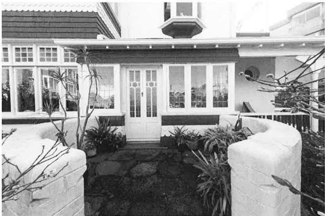
Figure 9: Detail of Inter-war period sunroom to ground floor (enclosing part of the original verandah) south elevation "Lansdowne"
