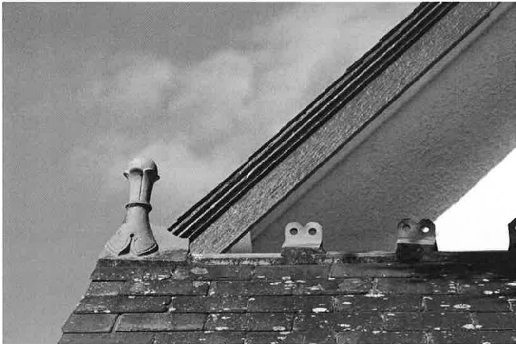
Figure 24: Ridge capping detail "Lansdowne"
