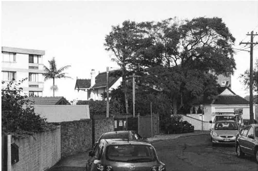
Figure 7: View of "Lansdowne" with east and north elevations visible (centre, slate roofed house to the left of the trees) from the east in Anderson Street. This view also shows the context in Anderson Street.
