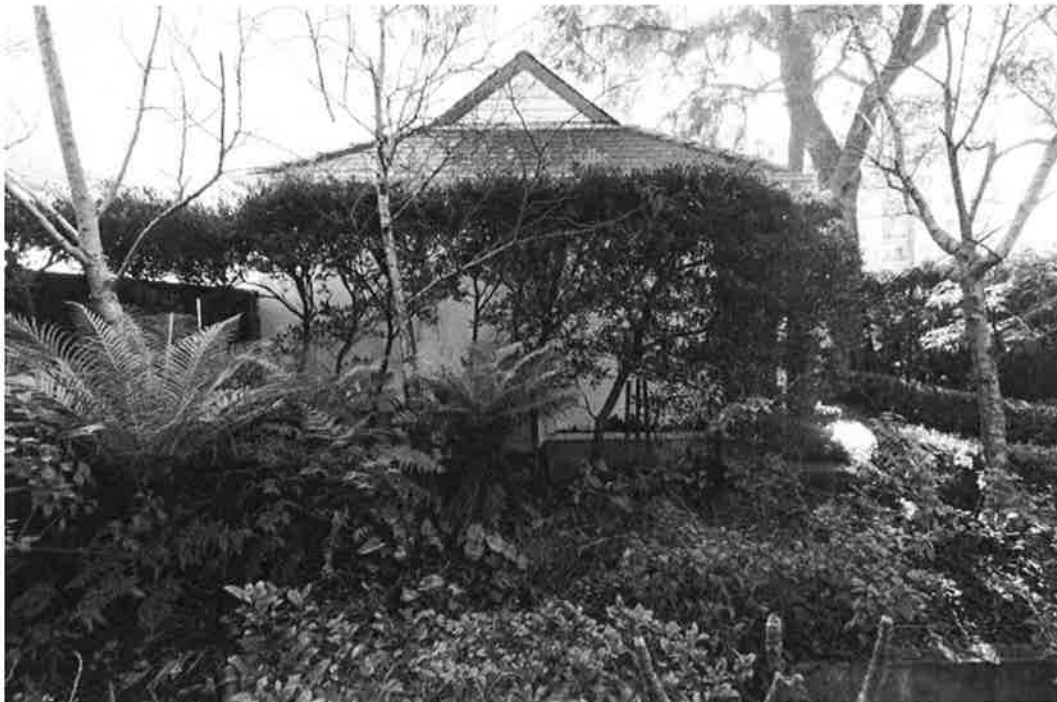
Figure 27: South elevation of the garage from within the garden, "Lansdowne"
