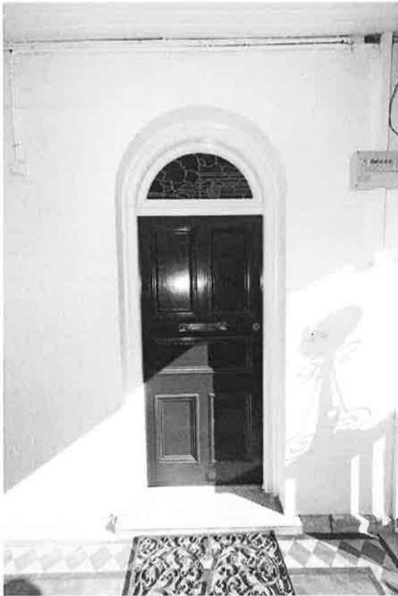
Figure 22: (Left) main entry door off the east verandah, Note semicircular leadlight fanlight.
