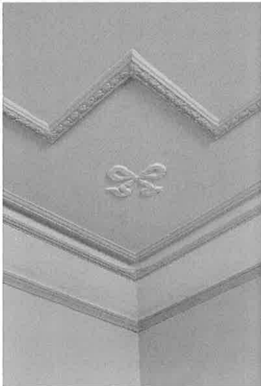
Figure 71: (Left) cornice and ceiling detail, first floor bedroom to the south-west corner of the house
