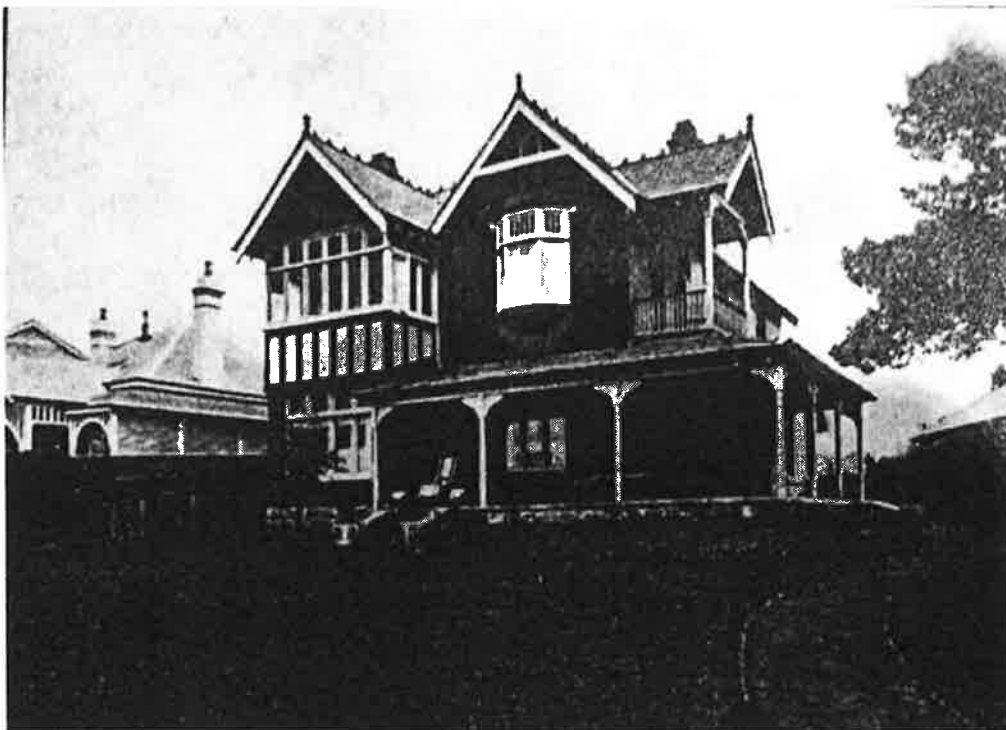
Figure 5: 1919 photo of the south (original front) and east elevations of "Coruisk" (later "Lansdowne") at No. 3 Anderson Street, Neutral Bay Source: Properties & Premises 1 September 1919, reproduced from Figure 9 of the GML Heritage Report on 3 Anderson Street, June 2014
