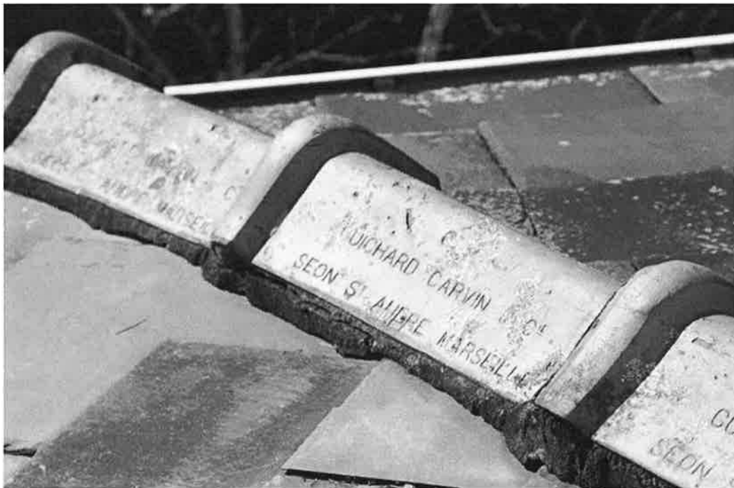
Figure 25: Terracotta ridge capping detail, "Lansdowne" with the Marseille (France) manufacturer's name
