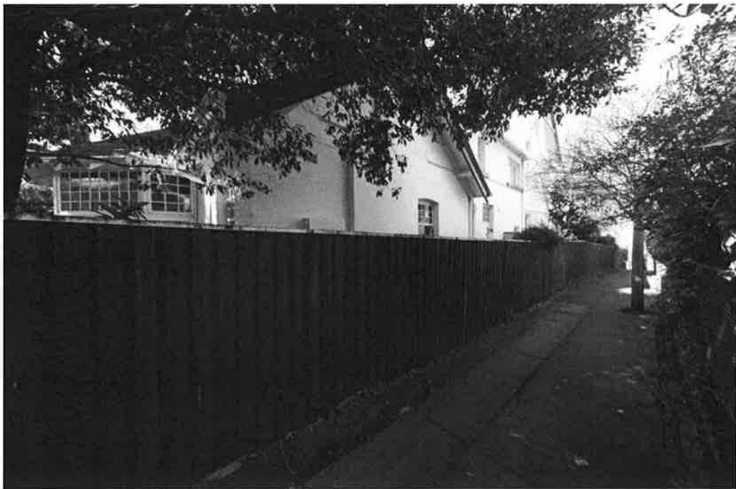
Figure 12: West elevation "Lansdowne" from adjacent public pedestrian laneway
